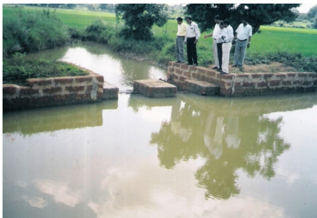
Fig. 4. Check dam for groundwater recharge
