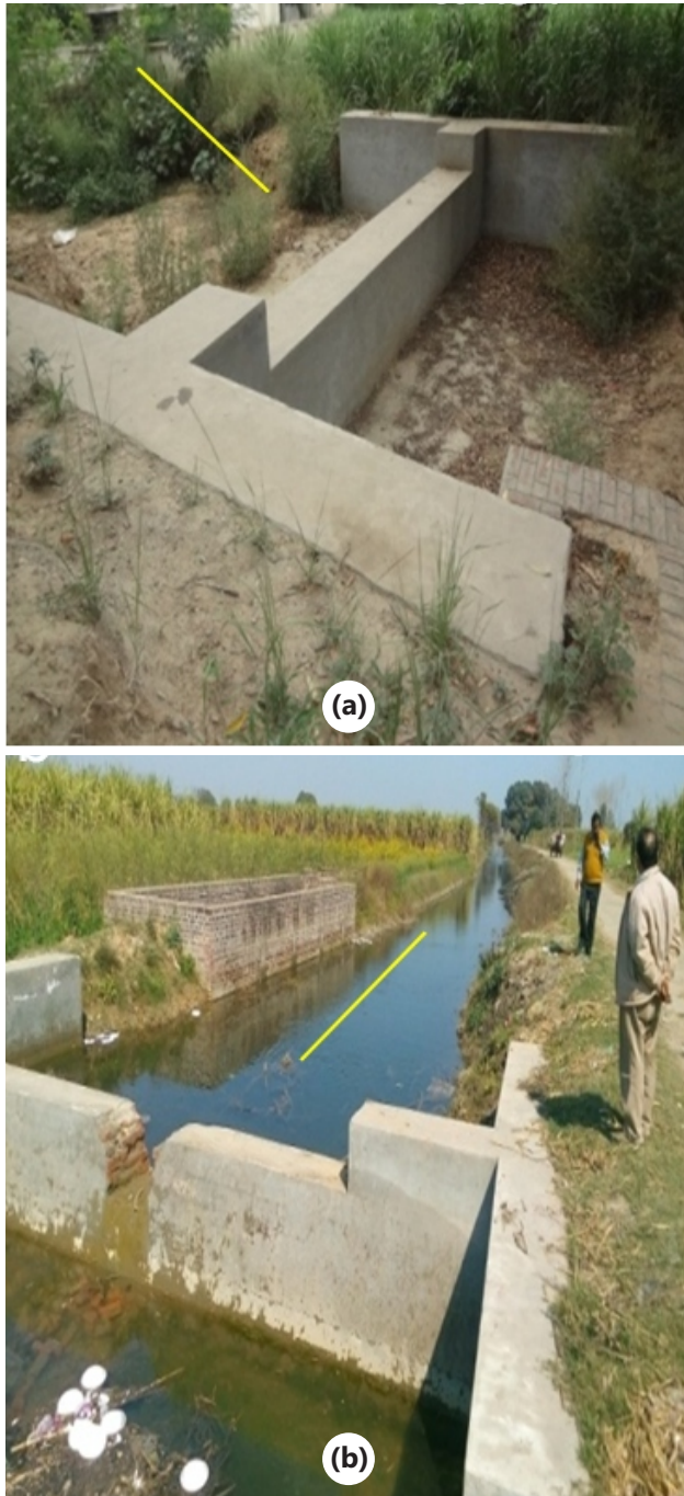
Fig. 3. (a) Overview of check dam WHS-I, (b) WHS II with water impounding in Harsauli drain of Rasulpur block, Muzaffarnagar district
