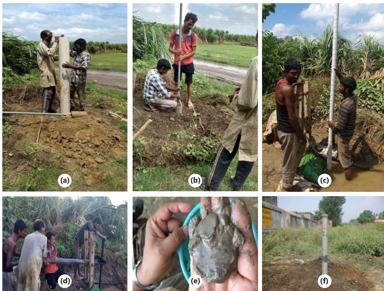
Fig. 5. Piezometer installation: (a & b) PVC pipe (2"dia) is placed in observation well, (c) 20 ft perforated pipe wrapped with fine filter net at normal pipe, (d) drilling operation, (e) observations of drill core material, (f) view of one of the installed observation well
