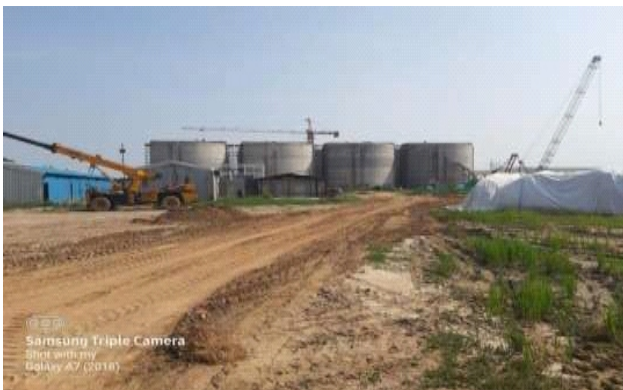
Photo 5. Digesters for producing biogas and bio-manure from bio mass and other organic wastes
