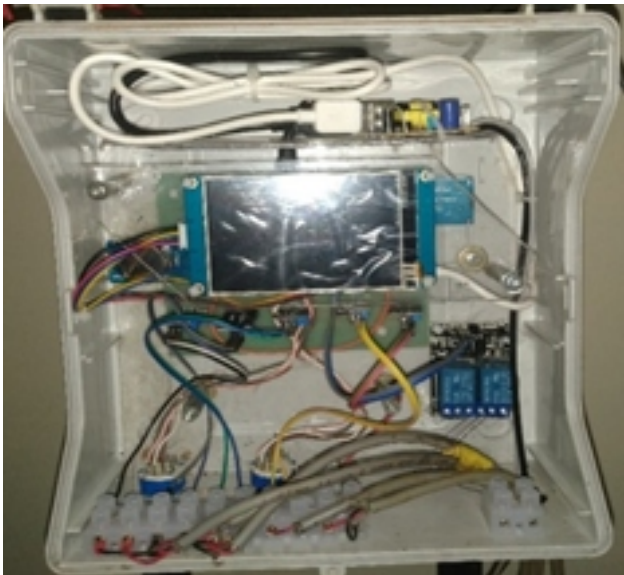
Fig. 6. Final assembled sensor system box
