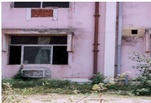
Fig. 5. Recharge pipe for rainwater collection
