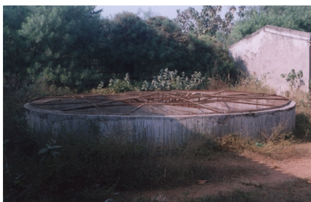
Fig. 6. Recharge dug well
